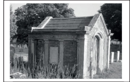
The newly re-roofed tomb
